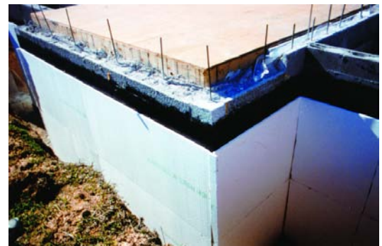
Basement wall with waterproofing and protective sheet
