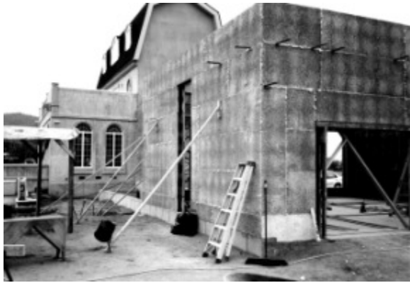
expanding the phase 1 home, with more ICF blocks
